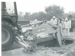
Water crew working on main line repair.
